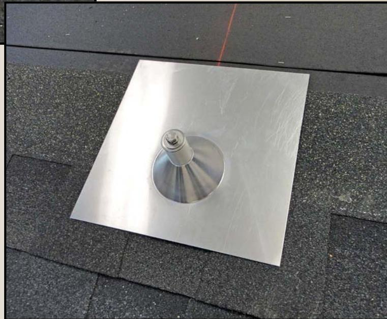
**Step 4 & 5** As the roofers work their way up the roof slope, they will install roofing material around the posts and install the appropriate flashing. This is a common practice, and similar waterproof flashing will be installed around vent pipes and skylights.
